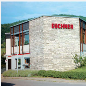
Production location in Unterböhringen
