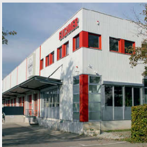
Logistics center in Leinfelden-Echterdingen
